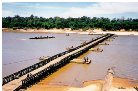
Fig. 4 – Bailey bridge (supported on unilocks). Source: [23].
